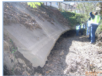
Middle: Eroded concrete creek bank.
