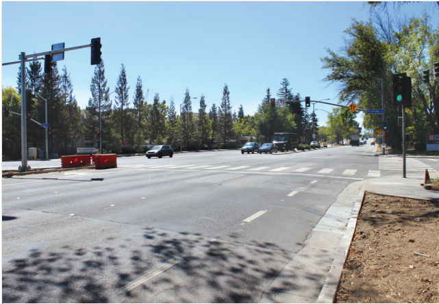
View 1: Looking South East on Wolfe Road.
