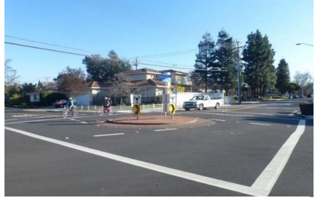
Figure 10. Traffic calming treatments help to reduce vehicle speeds and make walking safer and more
