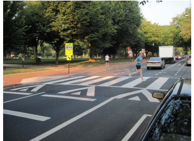
Figure 36. Raised midblock marked crosswalk
