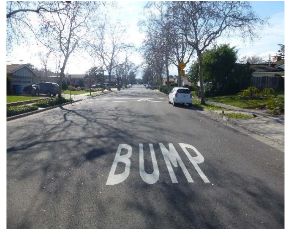
Figure 30. Speed hump, Cupertino
