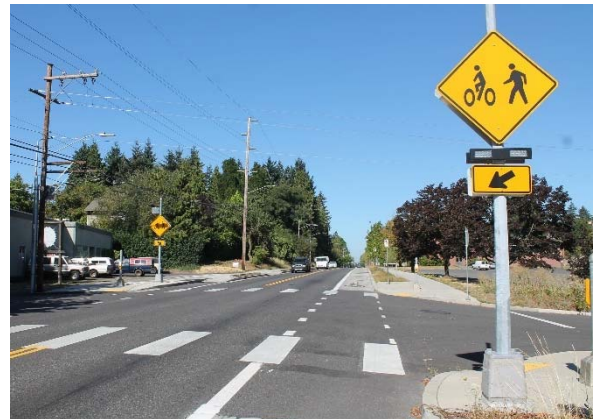
Figure 41. Rectangular rapid flashing beacon
