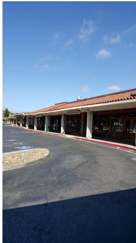
PHOTO #4. VIEW OF PARKING AREA.
