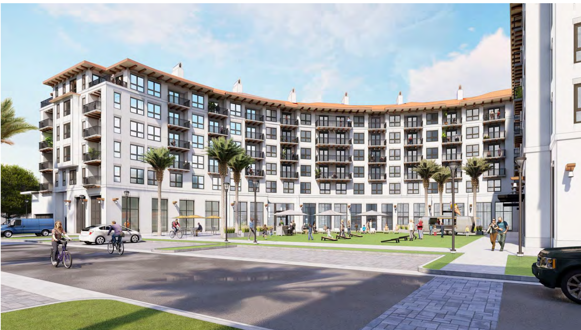
3/A210 - VIEW OF BUILDING 1 AT COMMON GREEN
