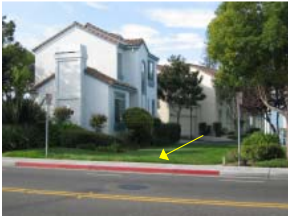
Fire access is marked where the fire truck can drive up over the curb across the turf block to access this housing development.
