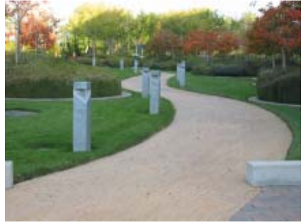
Permeable pavement and landscaped areas fill the courtyard on top of the parking structure.
