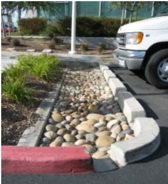
Rocky swale with curb cuts allows for infiltration to occur.
