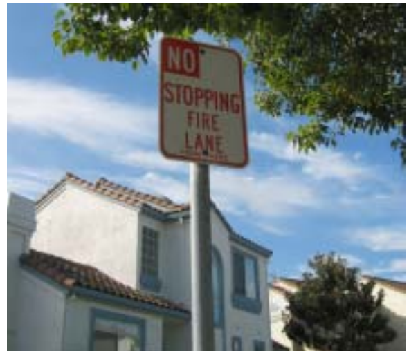
Signs clearly posted in order to prevent people from blocking access to the turf block fire lanes in emergencies.
