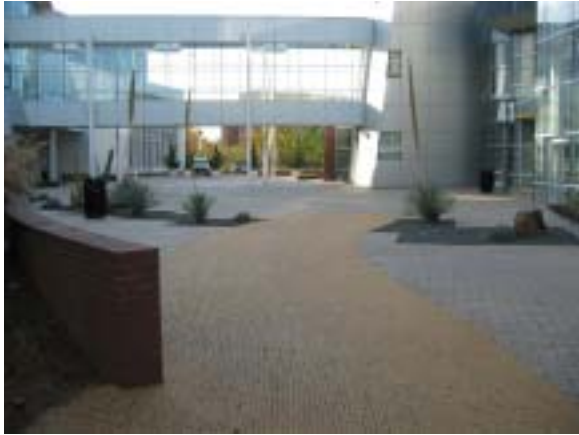
Permeable pavement is used in this courtyard.
